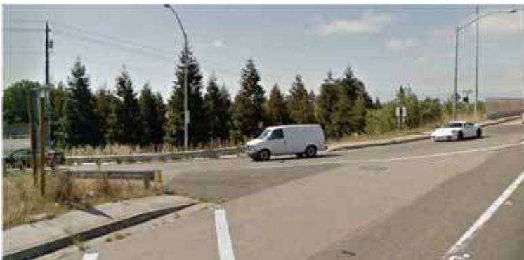
Figure 3-5: A missing crosswalk at a 20mph freeway on-ramp, Decoto Road and I-880
