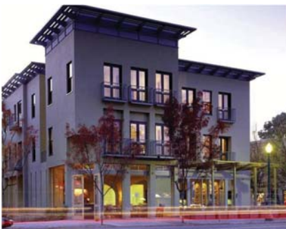
Special uses might include an educational or training facility (above), or hotel (below).
