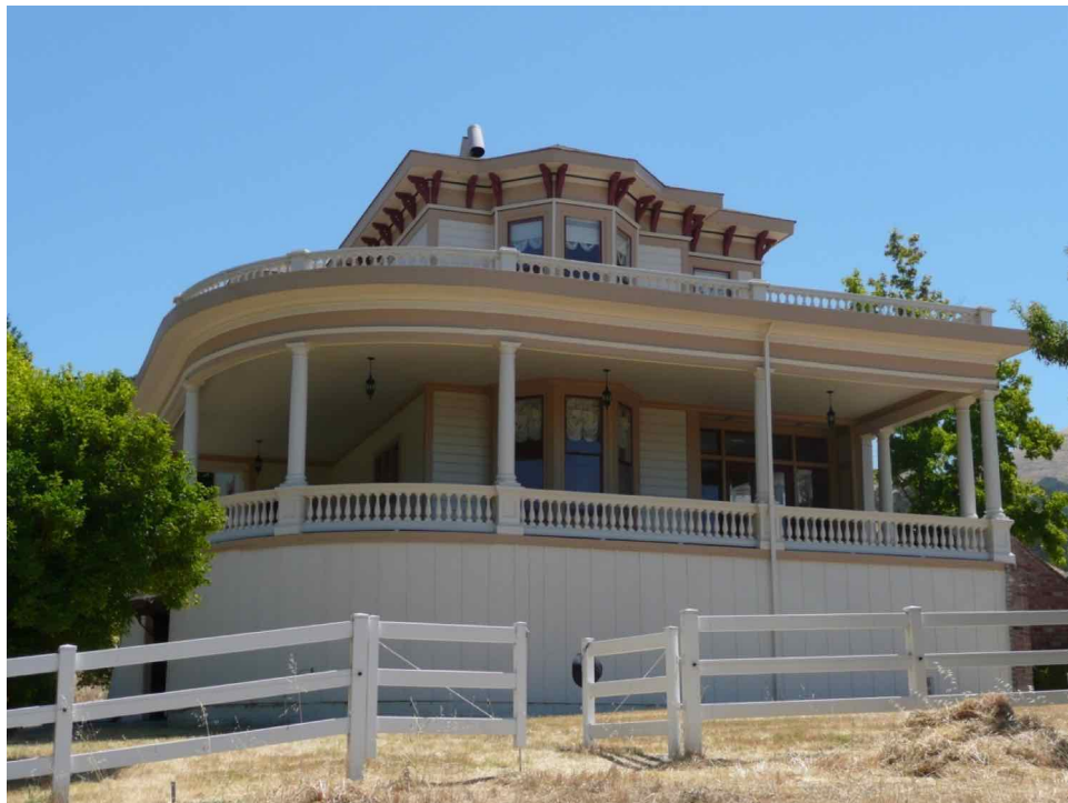
Figure 8: West elevation, showing veranda, facing east.
