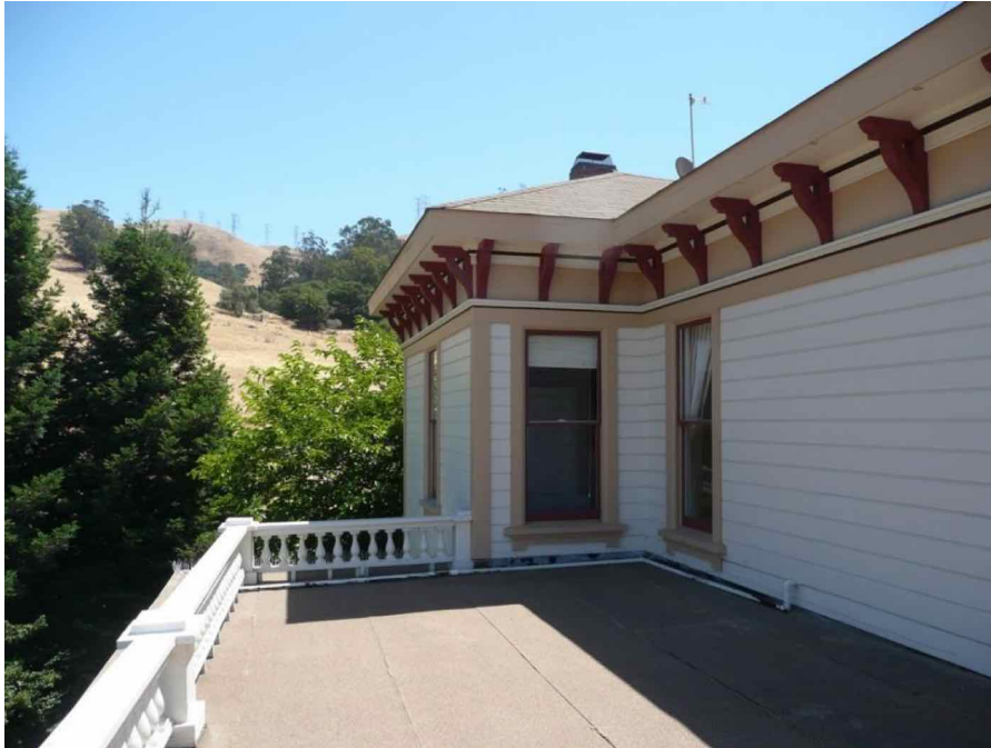
North elevation, showing second story fenestration from second-story porch, facing east.
