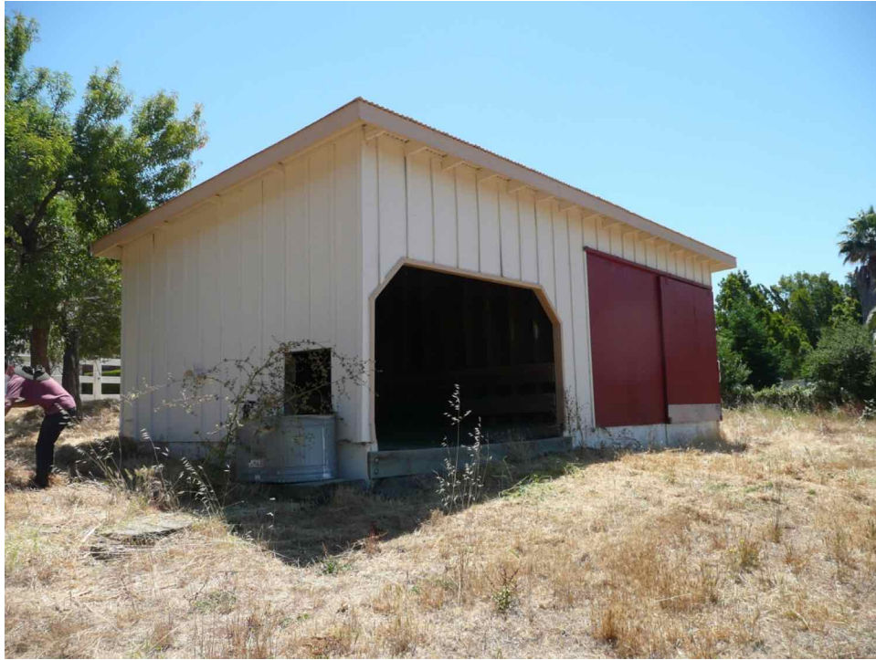
Figure 25: North and west elevations of contemporary horse tack building, facing southeast.
