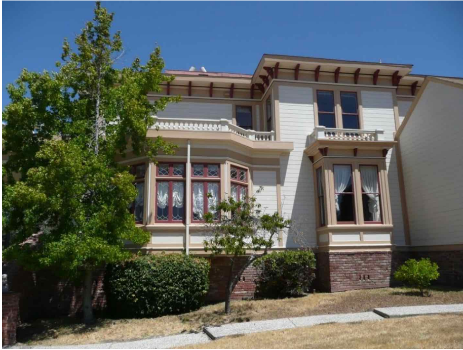
South elevation, showing ca. 1910 canted oriel bay at center-left and projecting bay at center-right, with gabled addition visible at far right, facing north.
