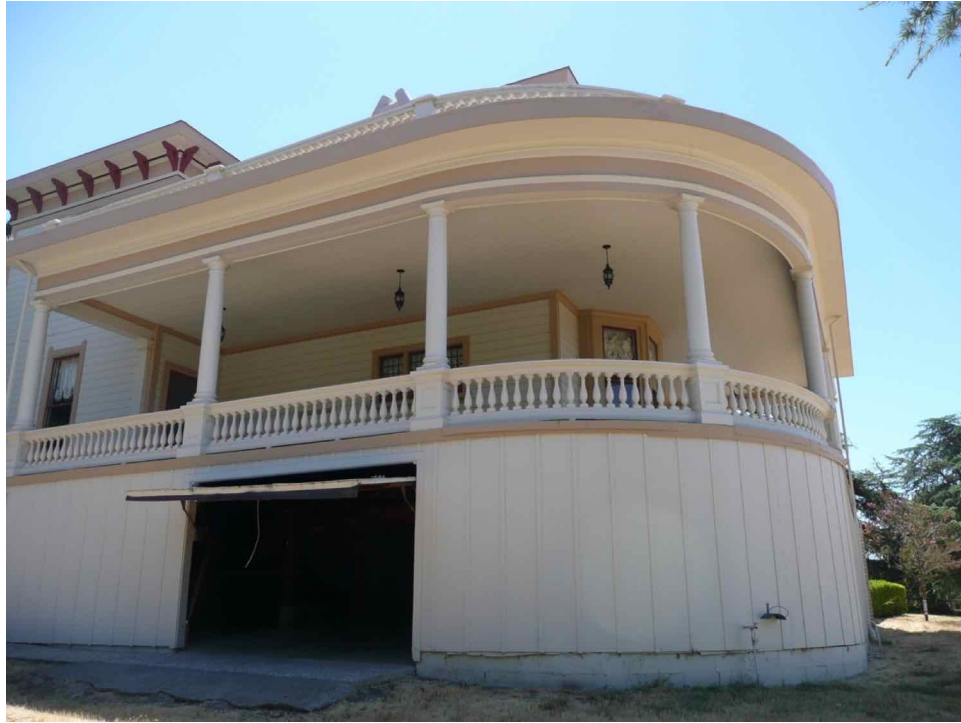
Figure 10: Wraparound veranda at north elevation, showing overhead garage door, facing southeast.
