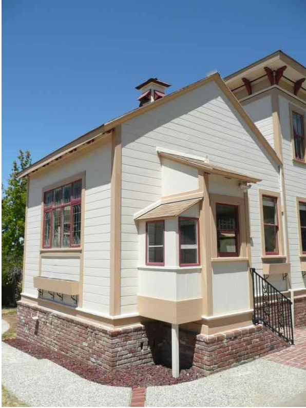
Gabled addition, showing south and east elevations with main two-story massing visible at right, facing northwest.
