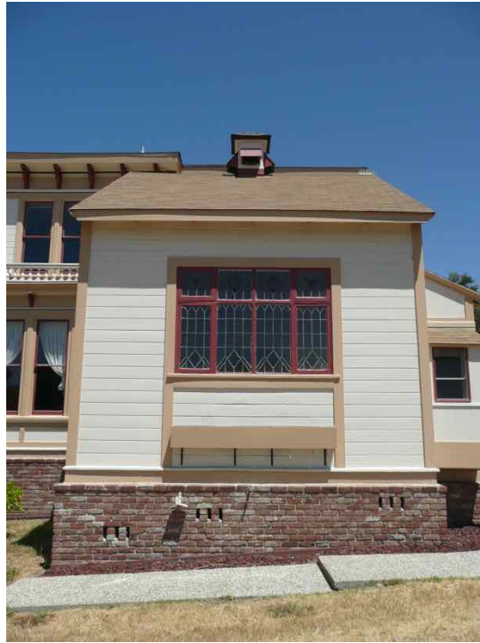
Figure 21: South elevation of gabled addition, facing north.
