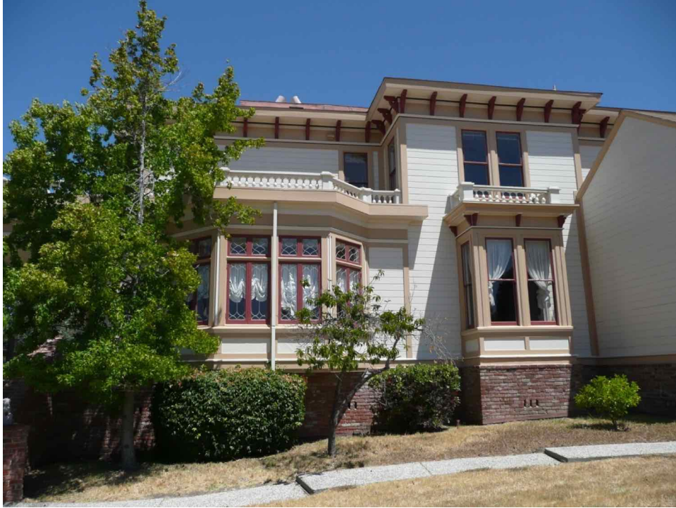
Figure 15: South elevation, showing ca. 1910 canted oriel bay at center-left and projecting bay at center-right, with gabled addition visible at far right, facing north.
