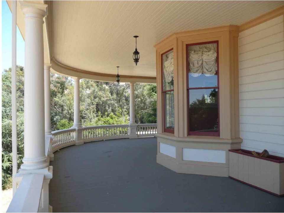
Figure 9: Bay window at west elevation from wraparound veranda, view northeast.
