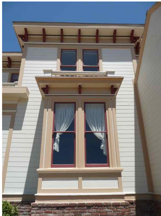
Figure 18: South elevation, showing fenestration at projecting bay, with gabled addition visible at far right, facing north.
