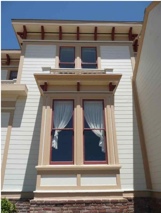
South elevation, showing fenestration at projecting bay, with gabled addition visible at far right, facing north.
