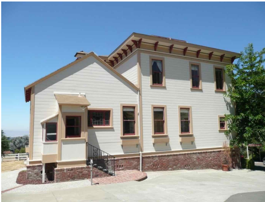
East elevation, showing gabled addition at left and main two-story massing at right, facing west.
