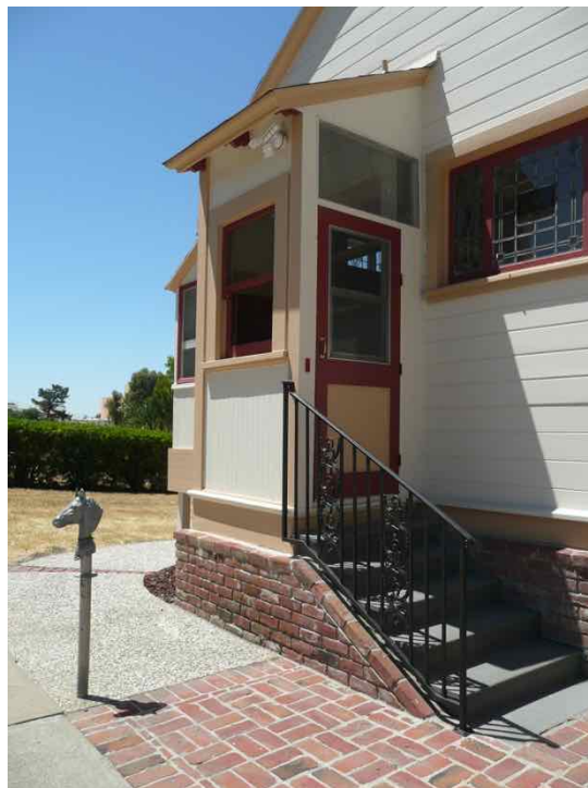
Figure 20: Early shed roof addition (rear entry portico) at east elevation of gabled addition, facing southwest.
