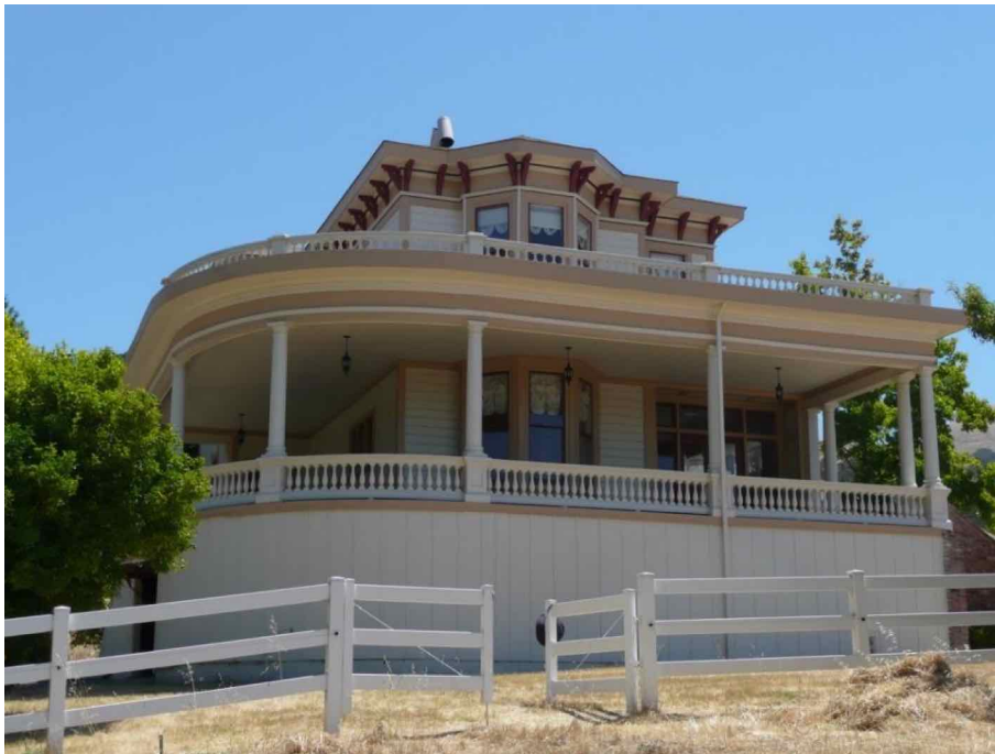
West elevation, showing veranda, facing east.
