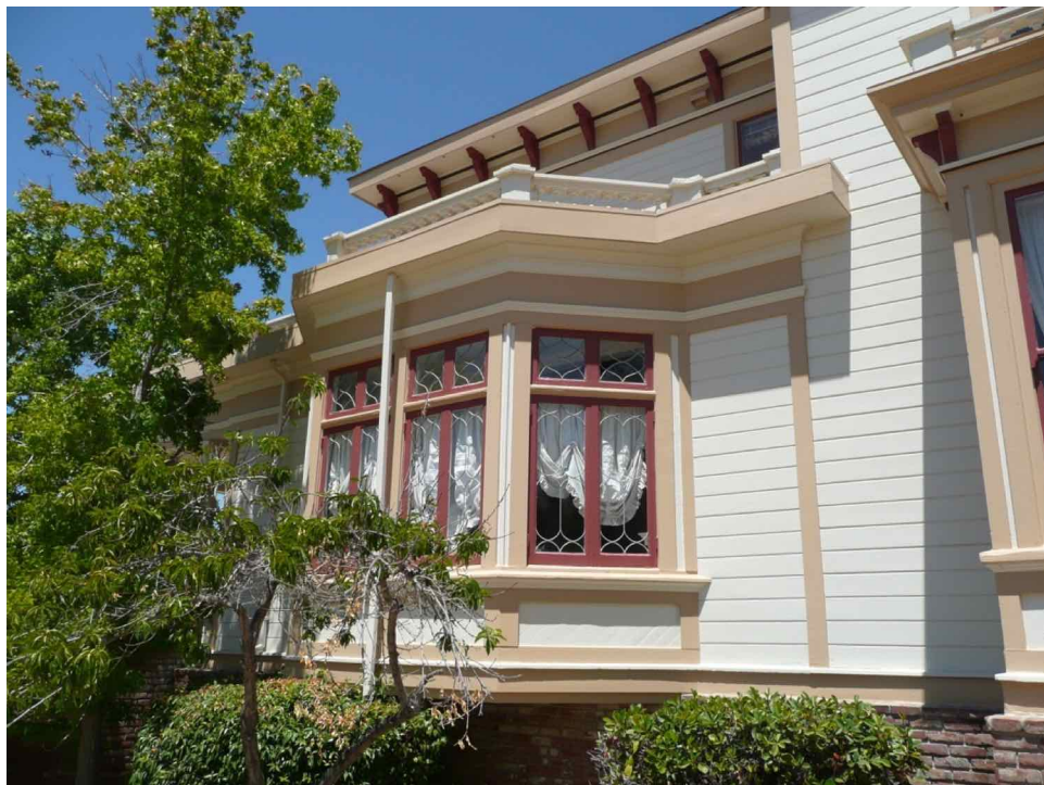
Figure 17: South elevation, showing ca.1910 canted oriel bay, facing northwest.
