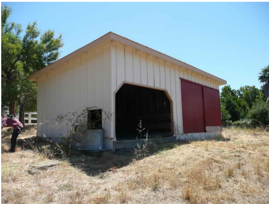
North and west elevations of contemporary horse tack building, facing southeast.
