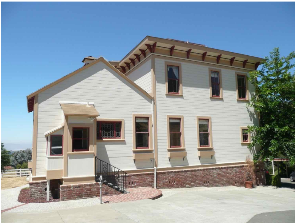
Figure 14: East elevation, showing gabled addition at left and main two-story massing at right, facing west.
