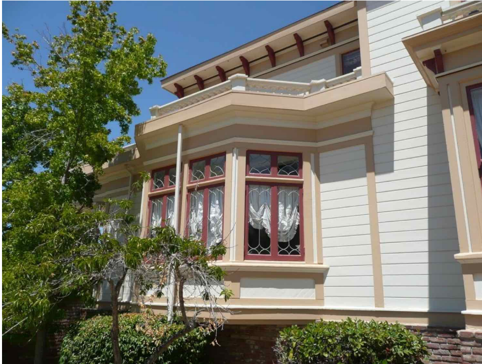
South elevation, showing ca.1910 canted oriel bay, facing northwest.
