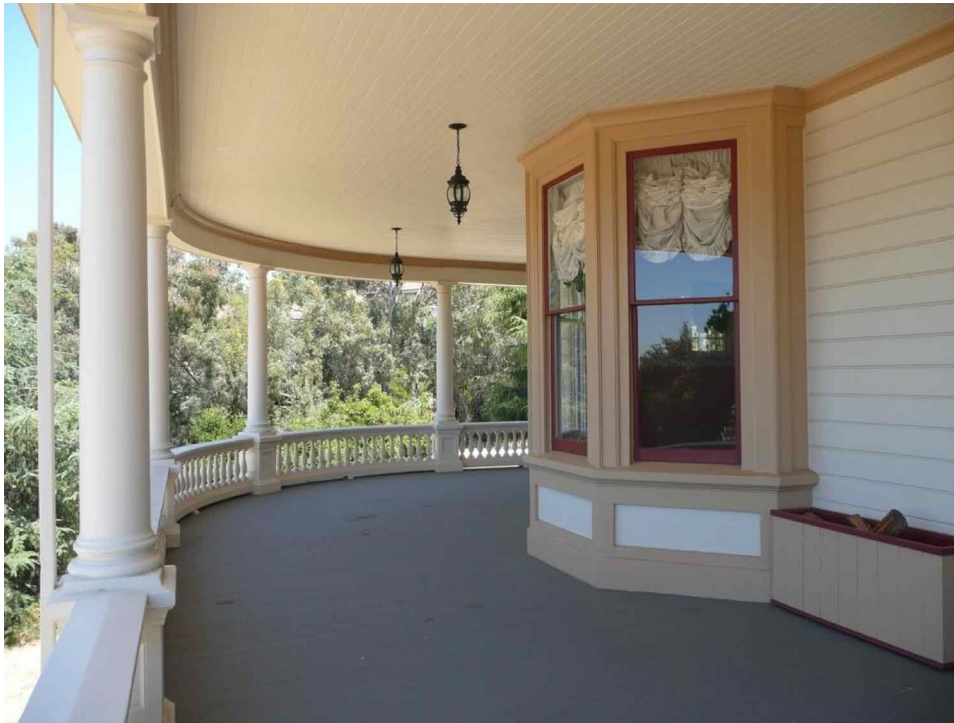
Bay window at west elevation from wraparound veranda, view northeast.
