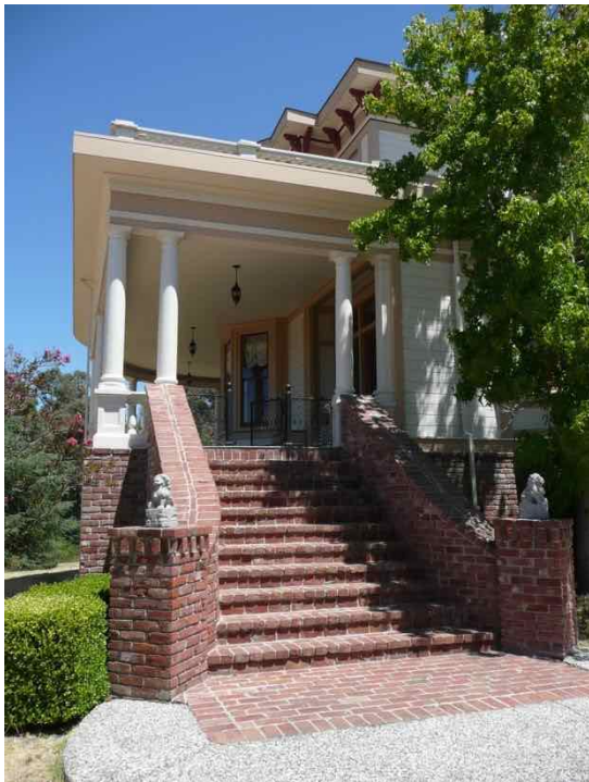
Brick entry stairs to wraparound veranda, facing northeast.
