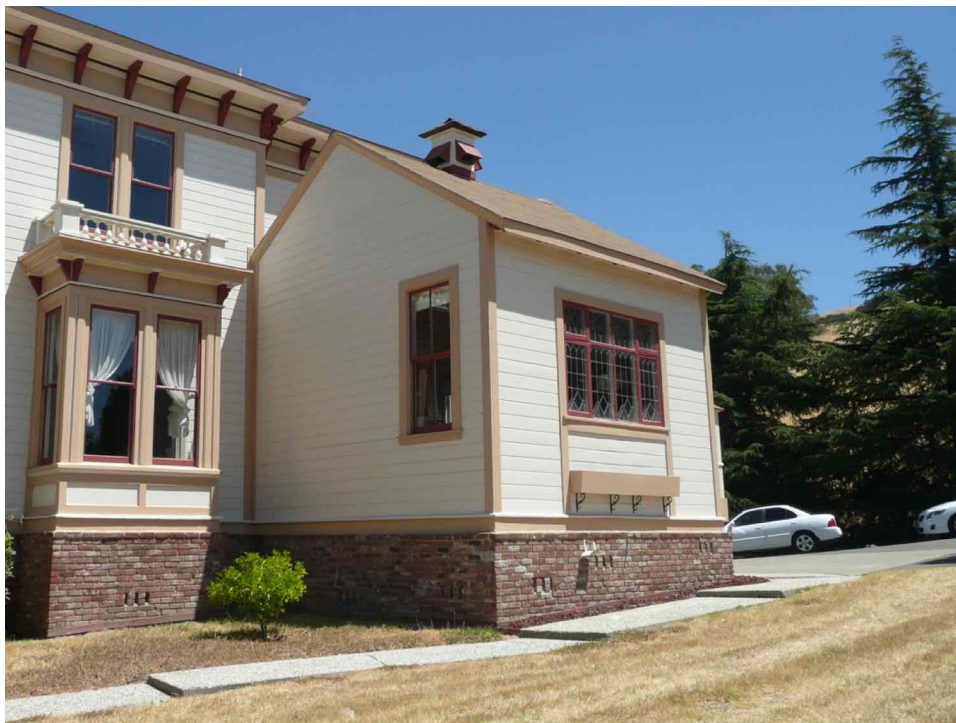
Figure 22: Gabled addition, showing west and south elevations with main two-story massing visible at left, facing northeast.
