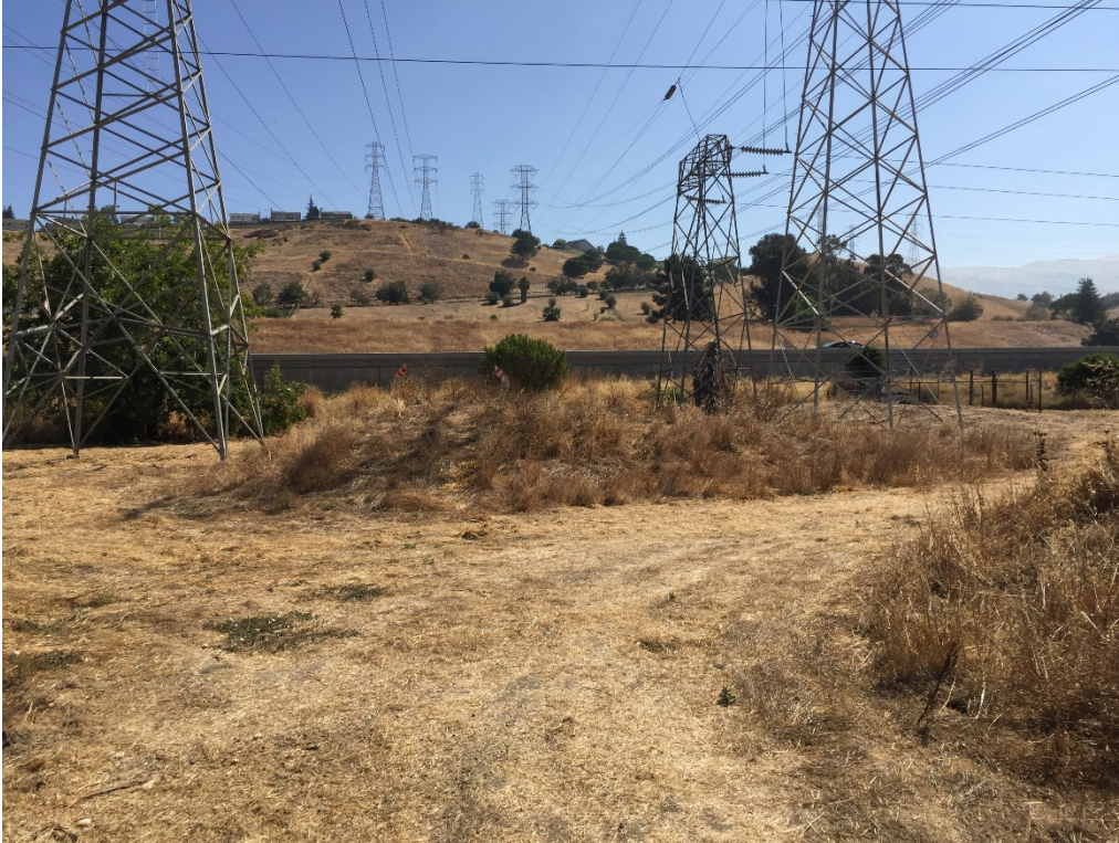
Photograph 2. Electrical transmission towers and soil stockpiles in areas not cleared.
