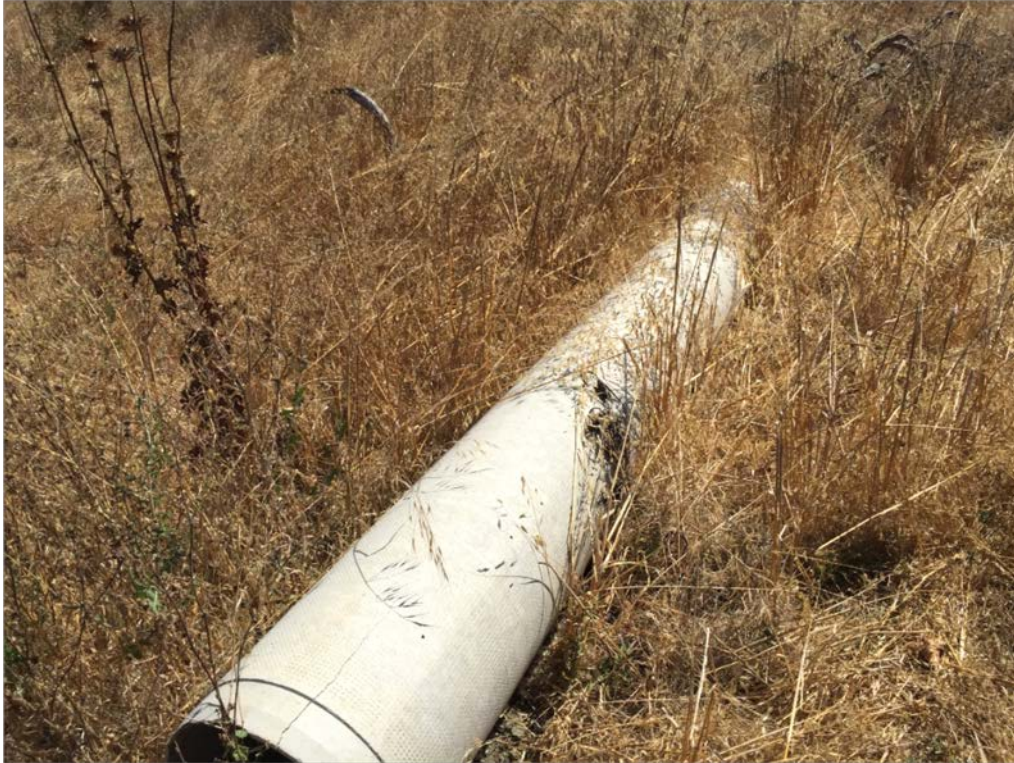
Photograph 10. Pipe (possibly asbestos cement) observed on Site.
