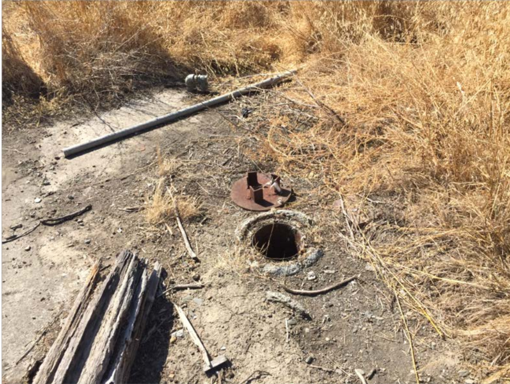
Photograph 8. Water well with cap removed and surrounding concrete pad.
