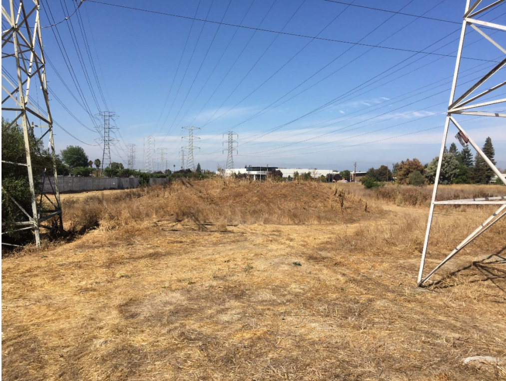
Photograph 4. Soil stockpile between towers.
