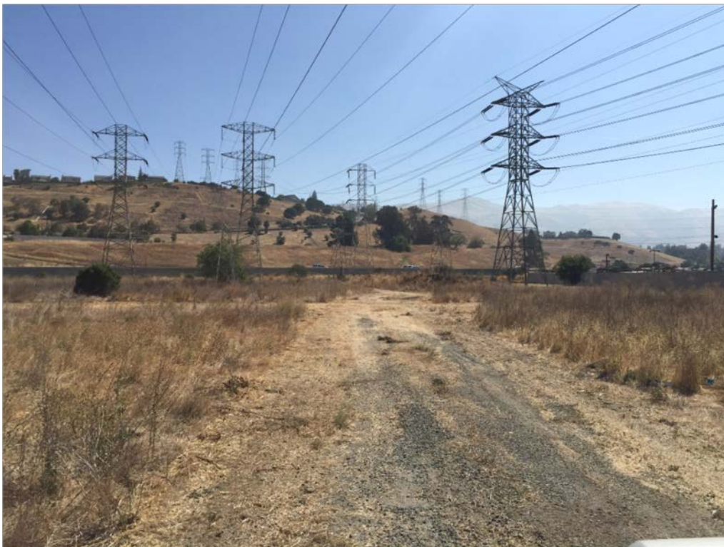
Photograph 1. Typical view of Site showing high voltage transmission towers and Cormack Road alignment.
