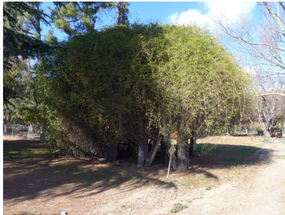
Figure 15: Water tank support structure (beneath vines)
