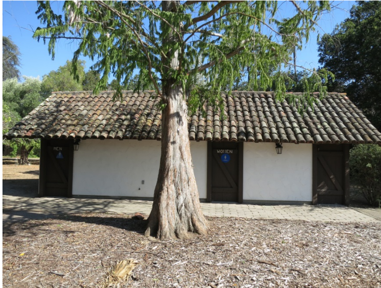
Figure 17: the Public Restroom and Storage Building.
