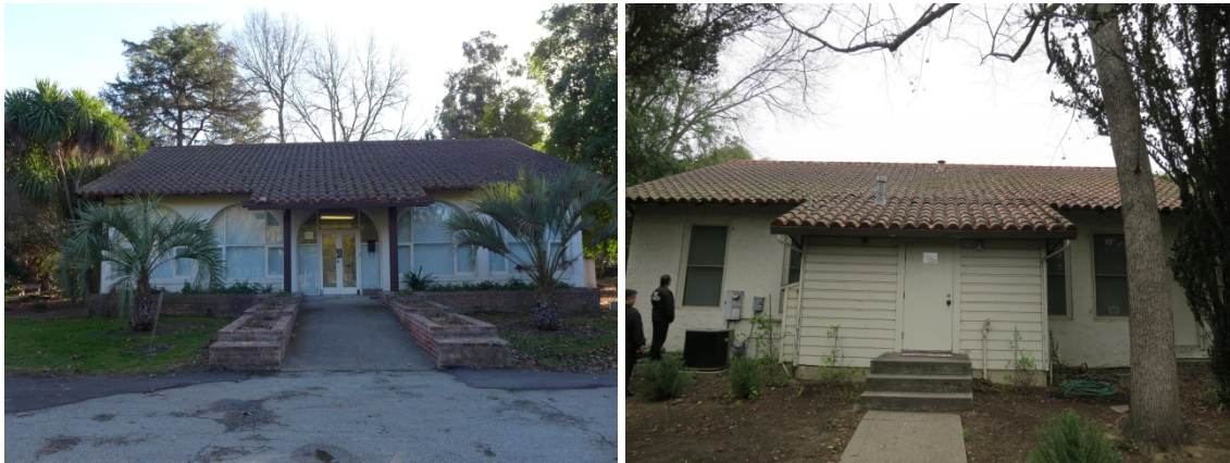
Figures 3 and 4. Nursery Office, front and rear elevations.
