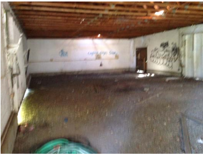
Inside shed from doorway
