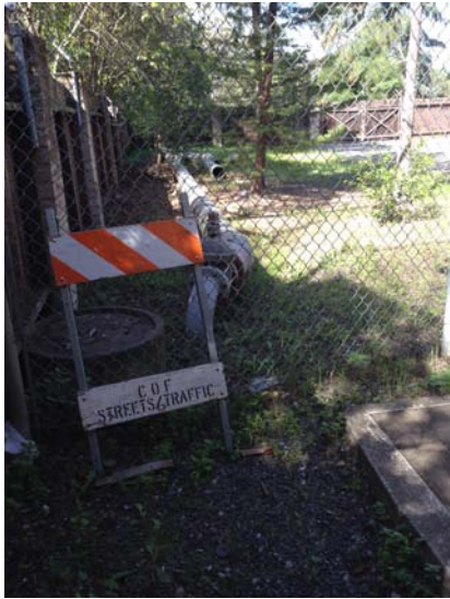
Pipe emanating from ACWD compound and going off-site
