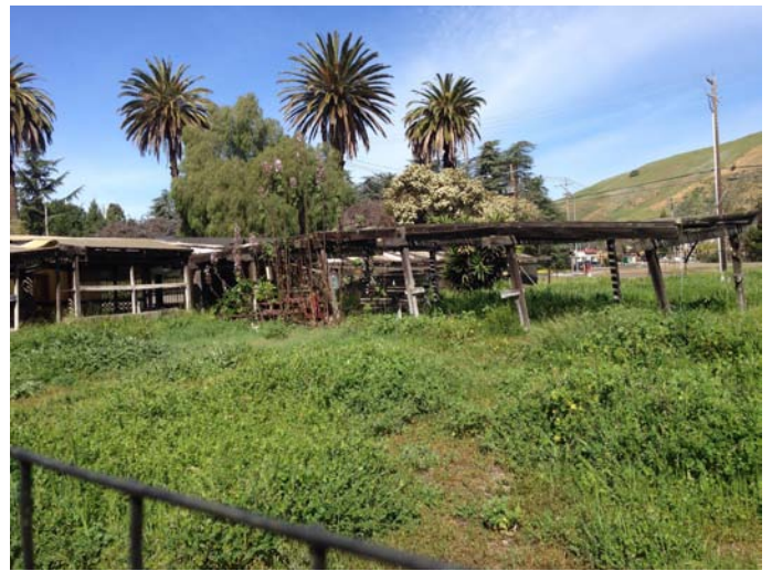
Looking toward entrance and abandoned structure (unsafe to access)
