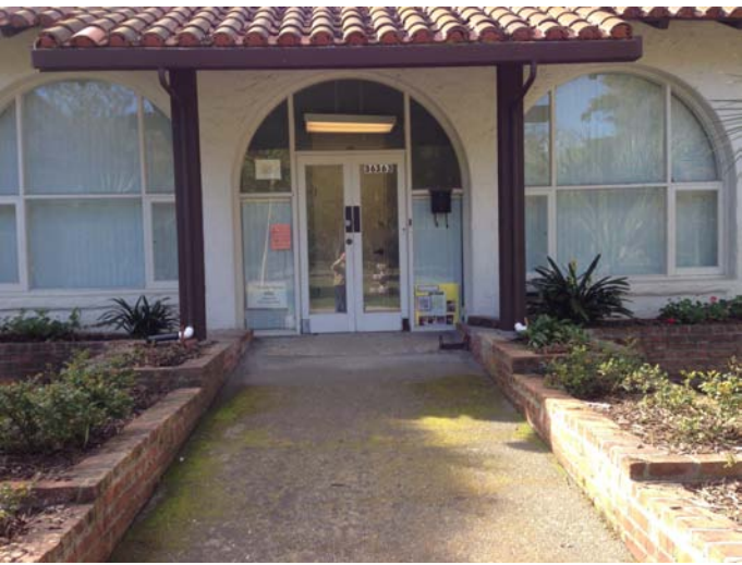
Front of California Nursery Admin/Office Building (no access)
