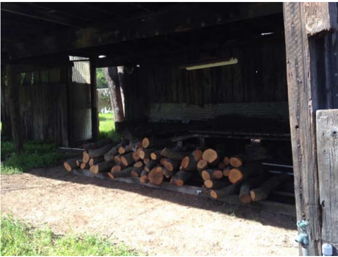
Eastern end of Packing Shed (no Access)
