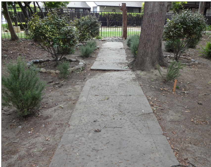
Photo c: Concrete walk on the south side of the office with a stipple finish and 6-inch band at the edge, 2014.
