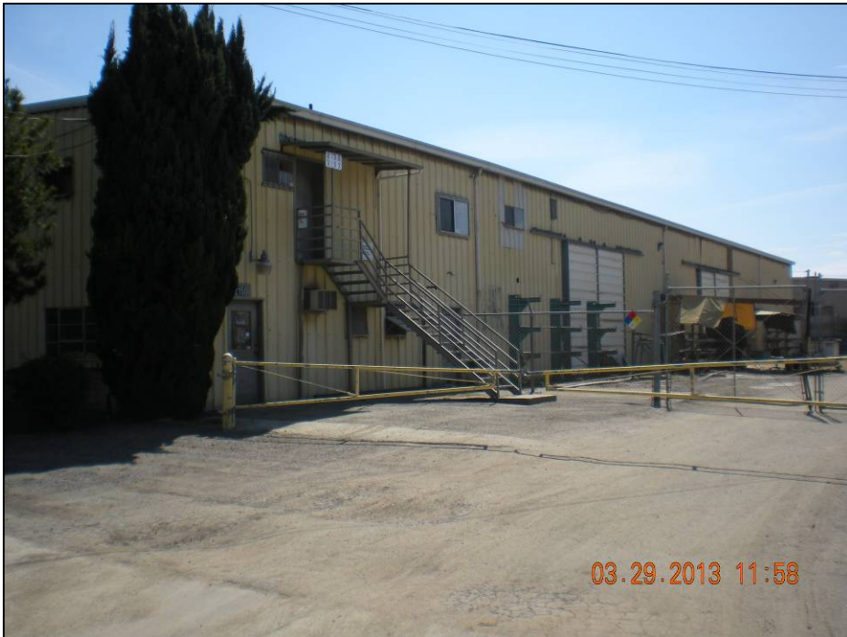
Photo 6: Typical view of older industrial warehouses located at 2150, 2152 and 2154 Prune Avenue.
