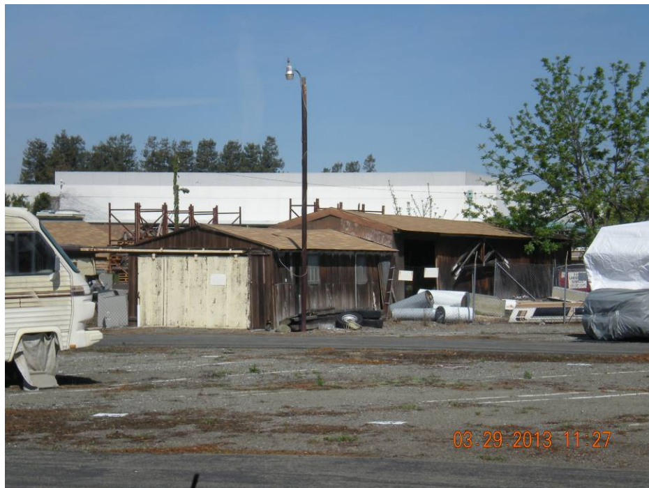
Photo 4: Typical view of older form farm buildings at 45946 Warm Springs Boulevard. Other similarly aged structures do occur on this property
