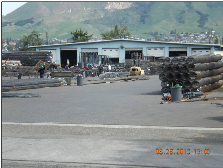
Photo 12: Commercial building at 45055 Fremont Boulevard.
