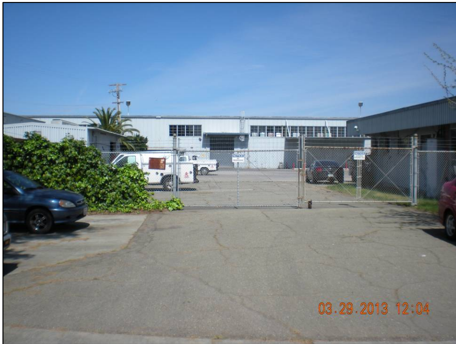
Photo 7: View of older industrial warehouse located at 2875 Prune Avenue bottling plant.
