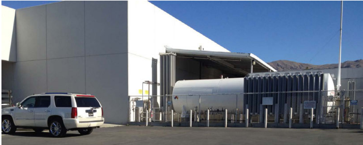
Figure 3: Example of Liquid Hydrogen Storage Tank in Study Area
