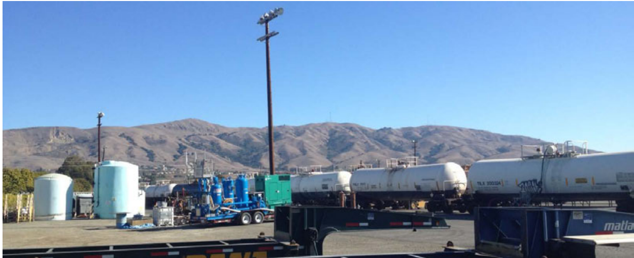
Figure 4: View of Liquid Rail Tanker Car Storage
