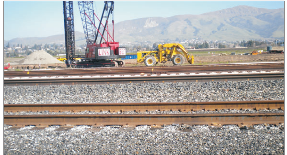
View of under construction Warm Springs / South Fremont BART station (January 2013).
