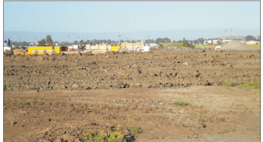
View of under construction Warm Springs / South Fremont BART station (April 2013).
