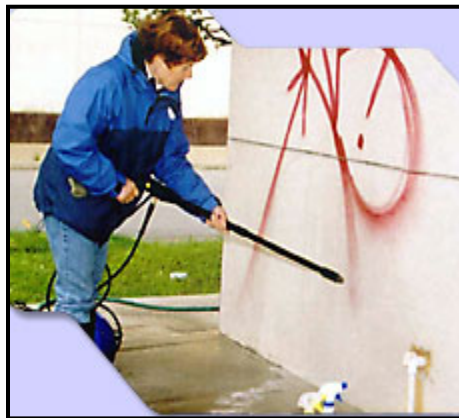
Figure 3: Fence Surface Treatment using paint, power wash and graffiti removal solvents
