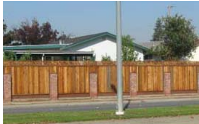
Figure 7: Existing Board on Board Style Fence along Blacow Rd.
