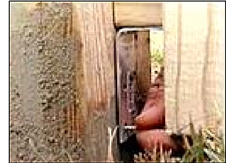
Figure B-2: L Bracket clamped to post
