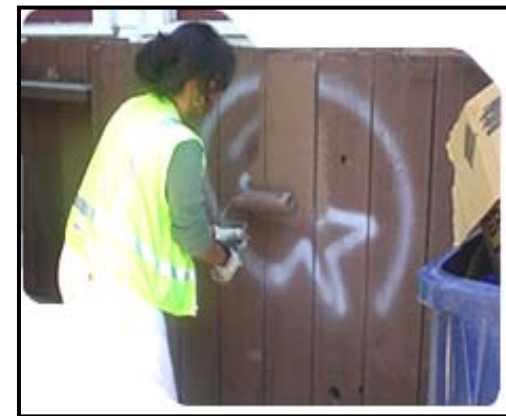
Figure 3: Fence Surface Treatment using paint, power wash and graffiti removal solvents
