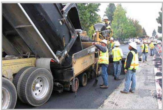
Street maintenance project
