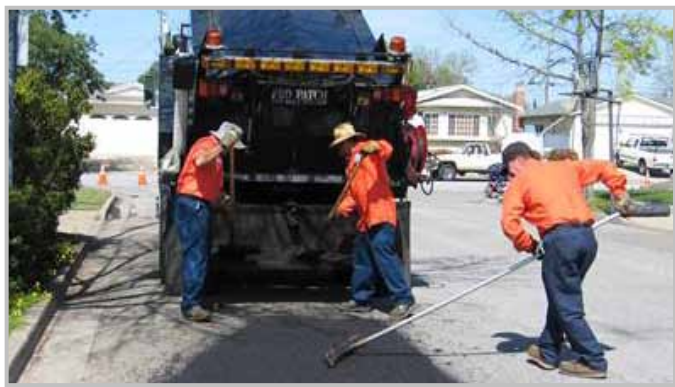
Asphalt patching in residential area
