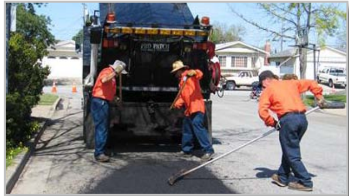
Asphalt patching in residential area
