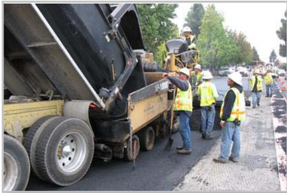
Street maintenance project
