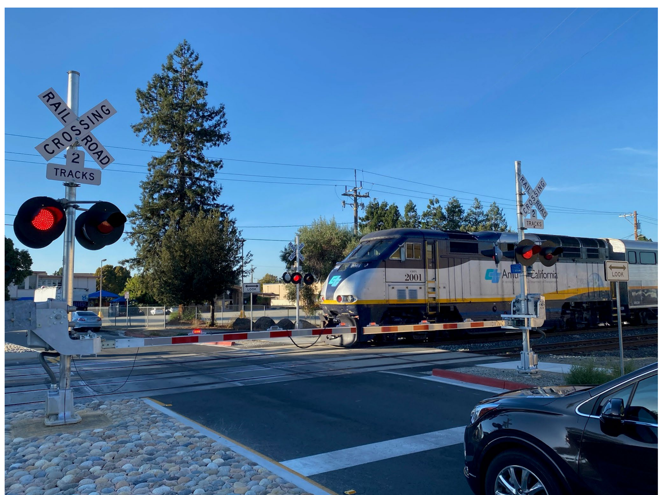
Photo of recently completed safety improvements at Dusterberry Way railroad crossing.
