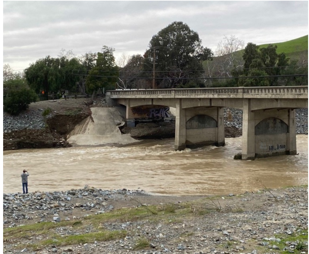
Old Canyon Road Bridge
