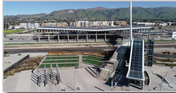
West Access Bridge
