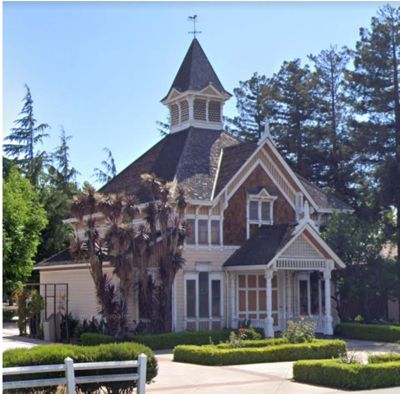
Historic Building Roof Repairs
