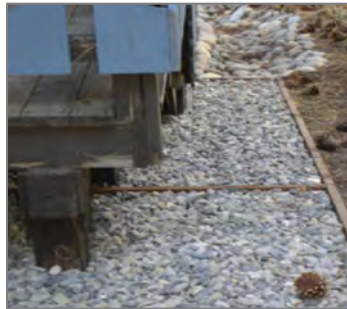
Gravel area under a gutterless roof
