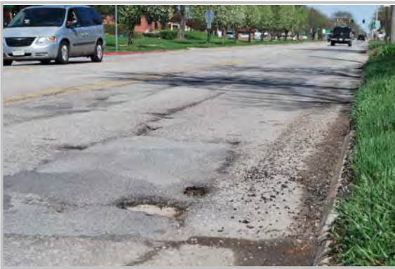
Street maintenance project
