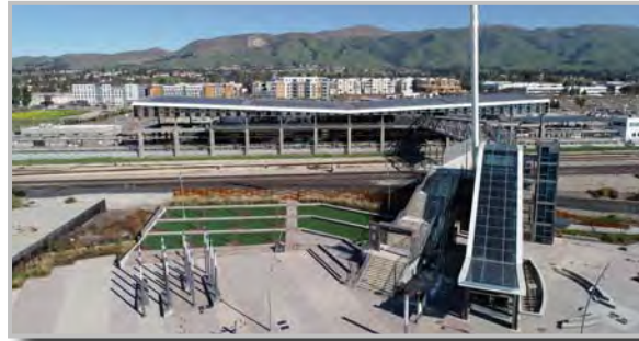
West Access Bridge
