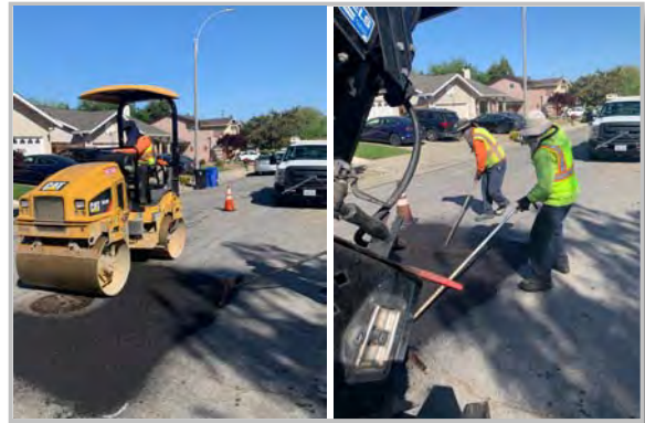
Asphalt patching in residential area
