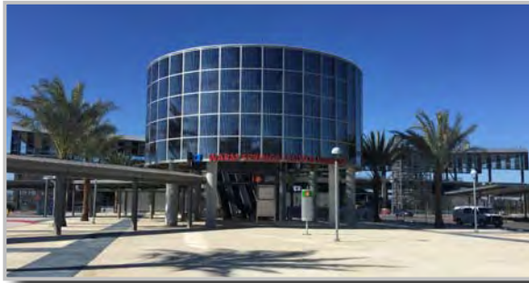
Warm Springs BART Station
