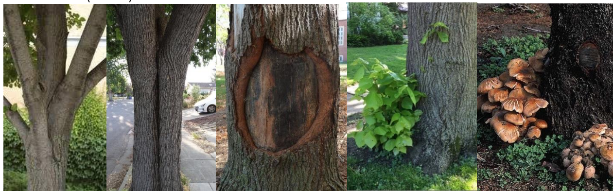
Image Description 24. Defects potentially impacting risk. From left: V-shaped branch unions, co-dominant stems, cavities and decay, sprouting (sucker) branches, and fungi (Armillaria root rot). Note: photos are not of Fremont trees
