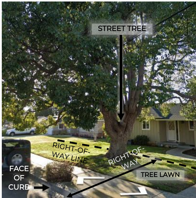
Monolithic Sidewalk – Sidewalk attached to curb
