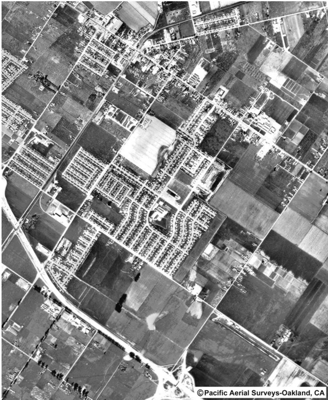
Glenmoor Gardens, March 2, 1958. More than 700 houses have been built in the subdivision, concentrated in the area above Blacow Road. The first two tracts have been laid out between Blacow Road and the Nimitz Freeway (I-880). (Courtesy of Pacific Aerial Surveys.)
