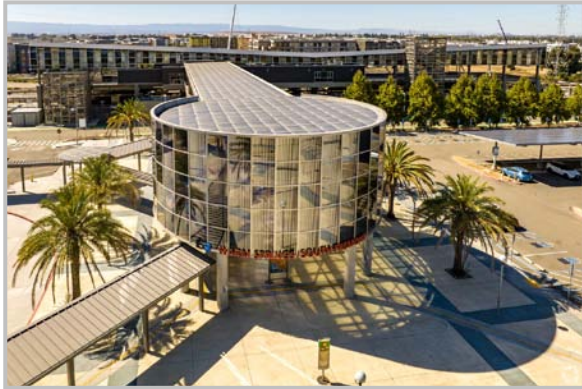
Warm Springs BART Station
