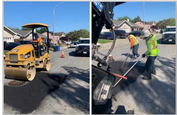
Asphalt patching in residential area
