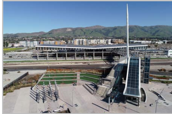
West Access Bridge
