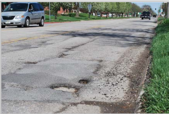
Street maintenance project
