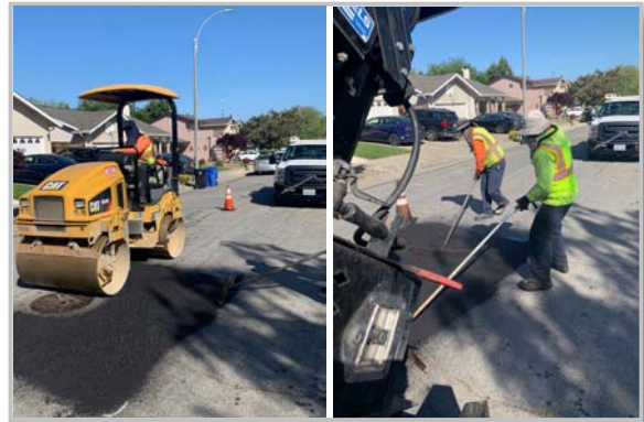
Asphalt patching in residential area
