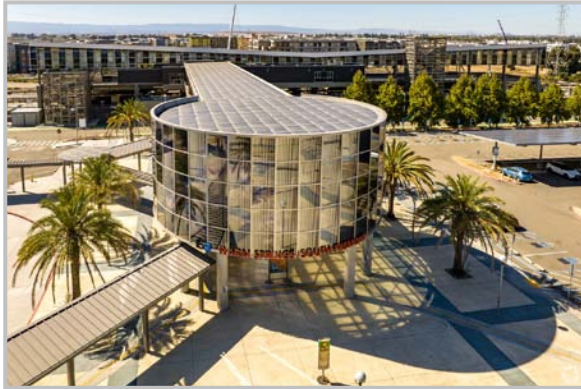
Warm Springs BART Station
