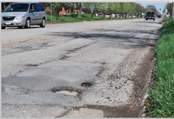
Street maintenance project
