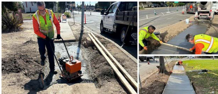
City crews replacing damaged sidewalks.
