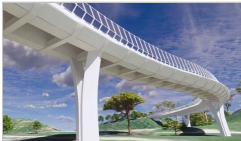
I-680/Sabercat Bridge and Trail
