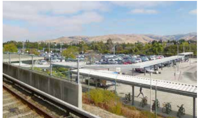
View of Fremont BART Station parking lot from south.
