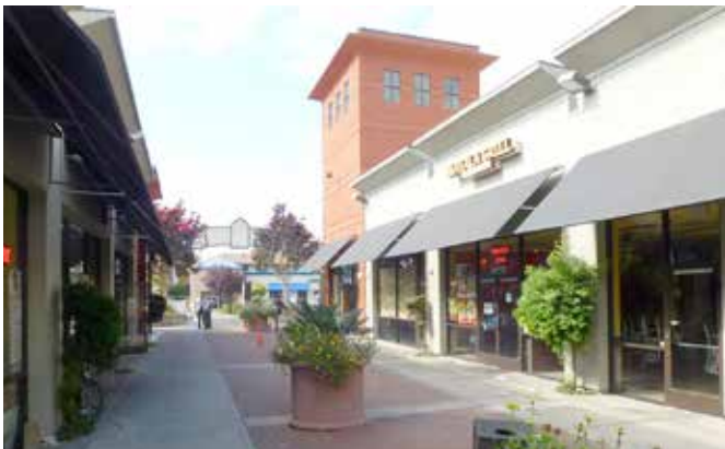
View of Gateway Plaza Shopping Center pedestrian passage
