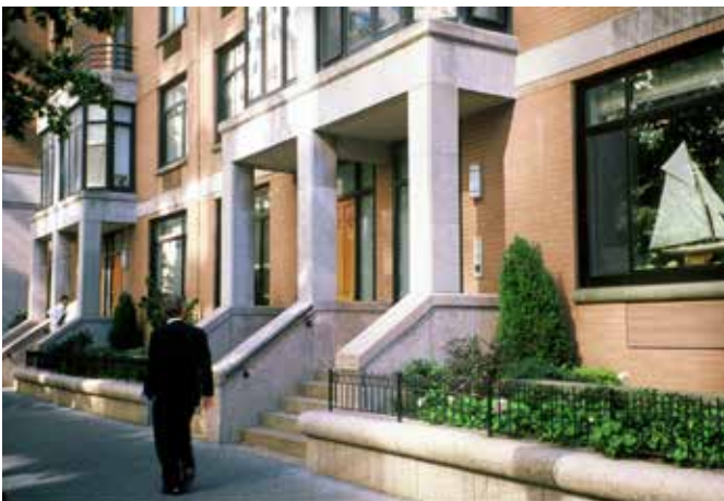
Stoop frontages can help contribute to a more urban character for Fremont’s City Center.
