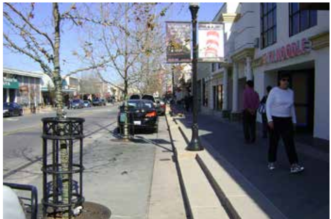
The City and developers need to be cognizant of existing storm drains when adding bulb-outs or moving curb lines.
