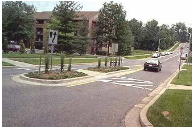
Bicycle lane and pedestrian island/crosswalk serve multiple user types. "Choker" island calms traffic in a residential area.
