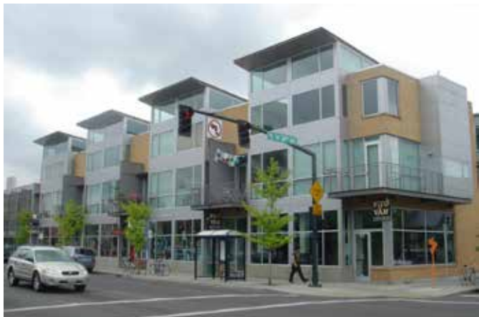
Pedestrian-oriented mixed-use building.
