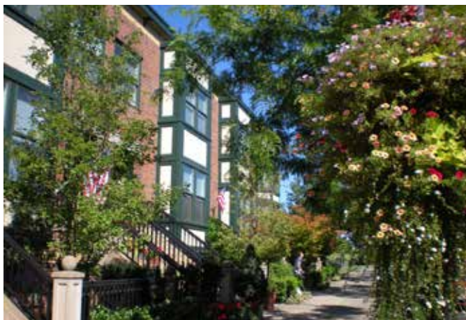
Multi-family housing facing a welcoming and comfortable pedestrian passage.
