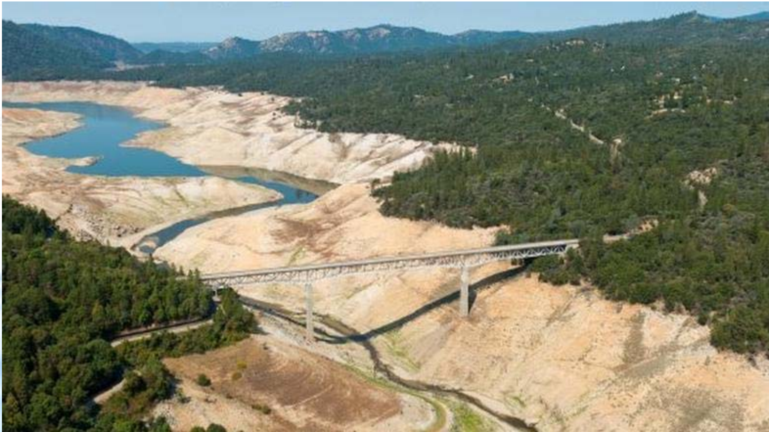
Lake Oroville in September 2015
