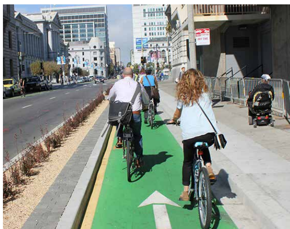
Example of protected bike lane (Polk Street, San Francisco).
