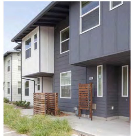
DON'T crowd uses onto a site. Design the setback transition zone to be adequately sized for activities. This zone is too narrow and does not leave enough room for any significant activity to happen.
