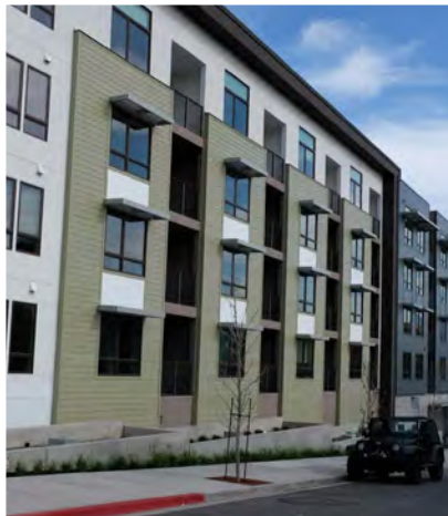
DON'T create flat façades. Provide depth between design elements. This façade looks flat with this composition. Awnings and paint do not create enough distinction between parts.
