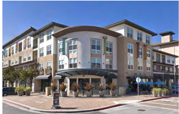
This vertical mixed-use residential building includes ground floor retail. The building corner is articulated with a lower, rounded volume and entrances that are easy to identify.
