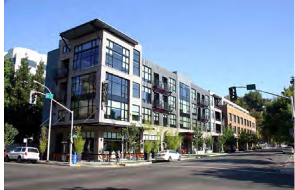
The appearance of larger buildings can be modified by using different façade materials, window rhythm, and roof lines to divide the building into distinct segments as seen from the street.
