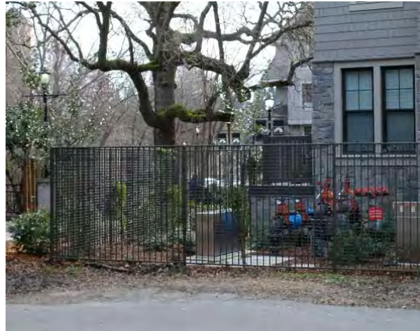
Locate utilities at the rear of building facades and behind fencing. Use vegetation and fencing to hide utilities.
