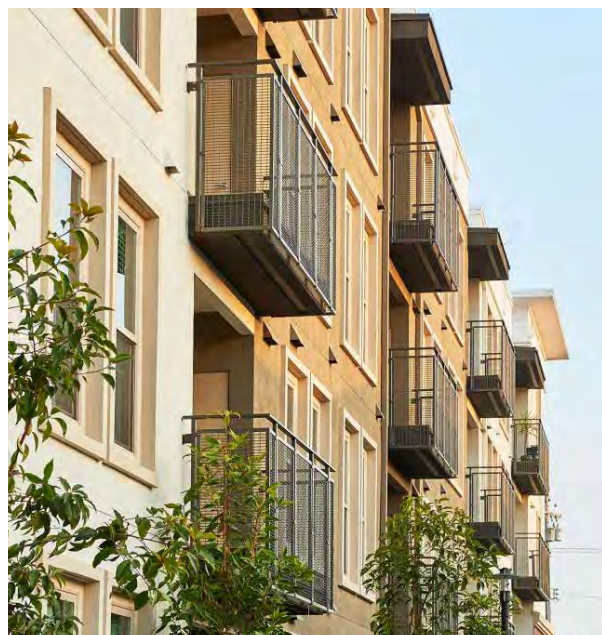
The expression of individual units using a pattern of overhanging and inset balconies makes the building function appear more "legible".
