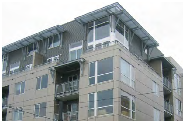
Example of top floor step-back.
