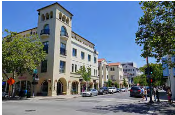
The massing of this vertical mixed-use building includes a tower feature on the corner. Its design distinguishes the ground floor of the building from the upper floors. Depth is added to the facade by setting back the top floor and recessing windows.
