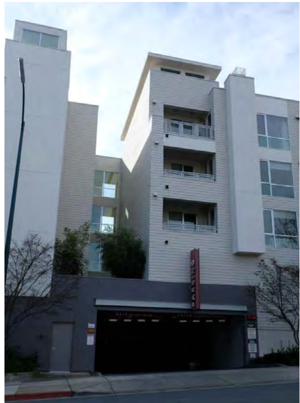
A minimally sized podium parking entrance located on a side driveway. The design of the parking podium is well integrated in the building with residential uses wrapped around it so that it cannot be seen.
