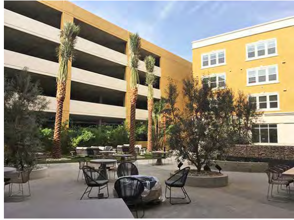
Open parking structure façades fronting common areas like one shown above are not allowed. Such façades must include screening elements.
