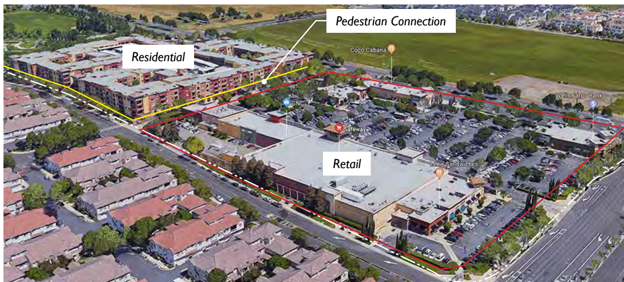
Retail and housing are mixed on this large site in a horizontal configuration.
