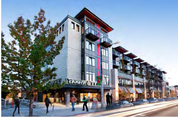
Vertical mixed-use buildings are often larger buildings. Careful building modulation and detailing can break down massing to an appropriate scale. Visual interest on facades typically utilizes three-dimensional detailing with cornices, window moldings, balconies, awnings, and reveals, to cast shadows and provide more articulation to the building mass.
