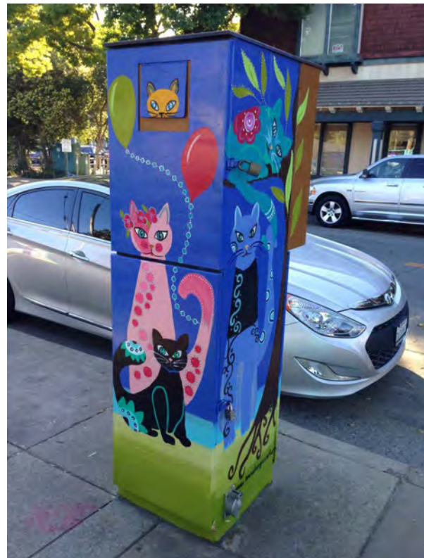
Paint existing utilities that cannot be moved.
