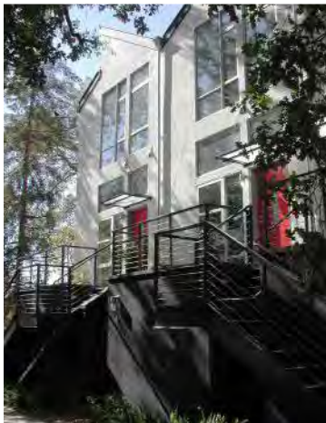
DON'T separate activity between the street and residential units with a full story feature. Stoops that transition half a level are acceptable.
