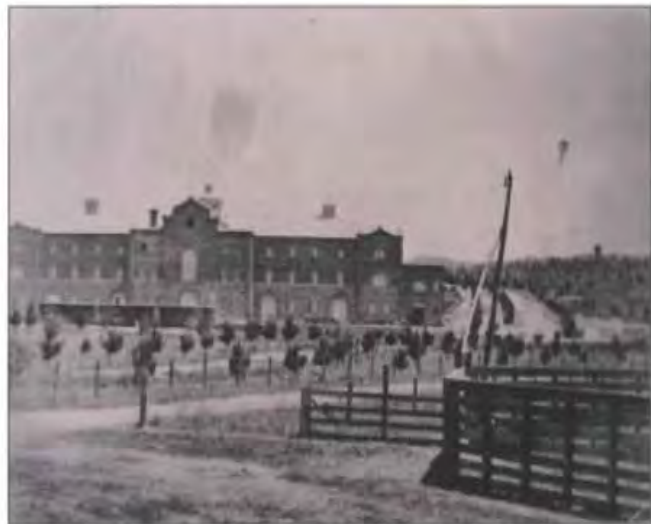
Photo 5. Gallegos Winery and grounds (Von Buskuh (?) pre-1906).
