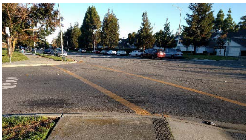
The southern Maybird Circle/Deep Creek Road intersection looking north.
