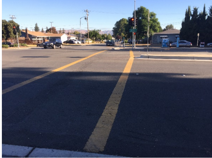
The Blacow Road/Boone Drive existing crossing.
