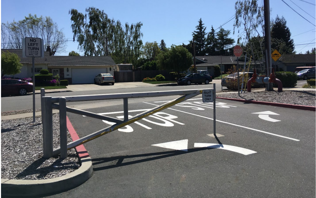
Swing gate at exit of drop-off loop discouraging left turns.
