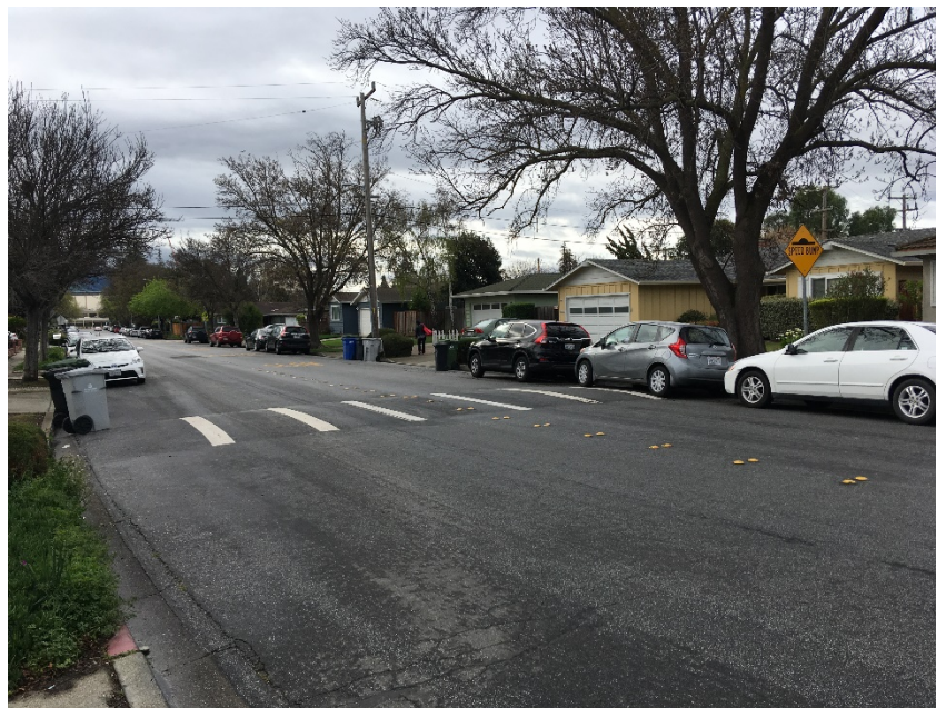
Speed hump with non-CA MUTCD compliant striping.
