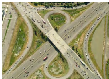
Caltrans maintains freeway intersections in Fremont.
