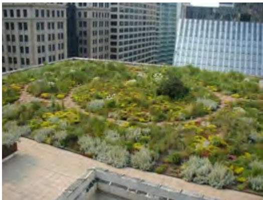
Urban Green Roof
