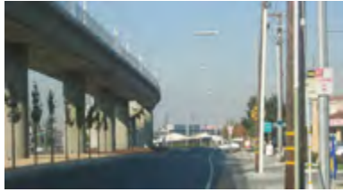
Neighborhood Barriers Elevated Rail
