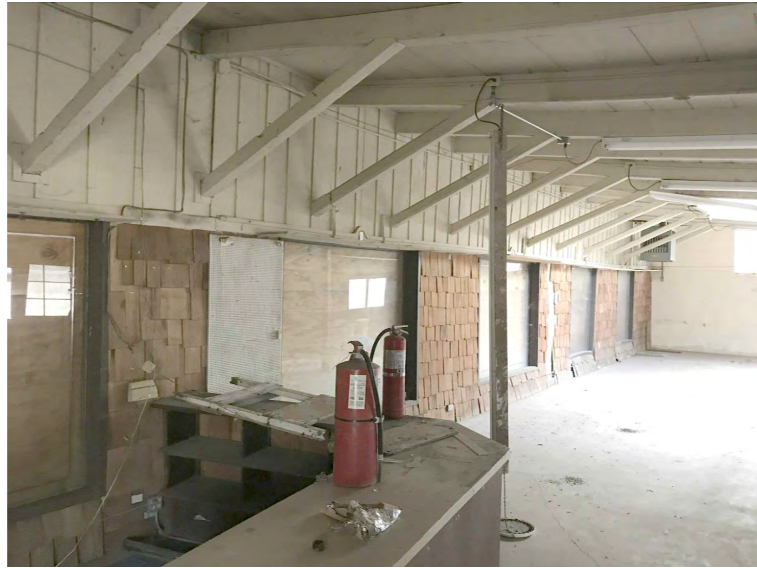
A INTERIOR - NORTH WING
