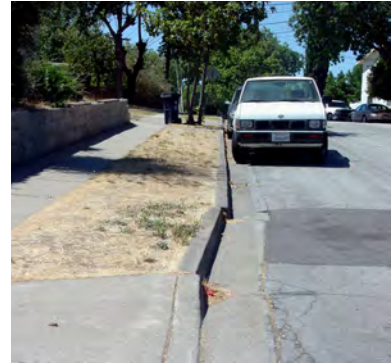
Evidence of fault creep in Fremont
