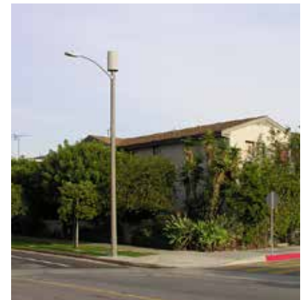
Copyright © 1997-2016 CellTowerPhotos.com. Used with permission.
