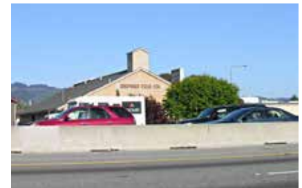
Copyright © 1997-2016 CellTowerPhotos.com. Used with permission.
