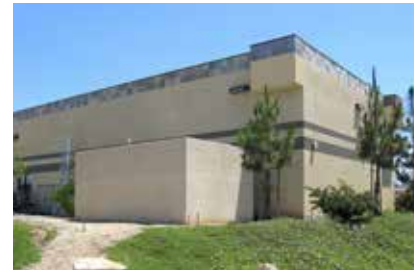
Copyright © 1997-2016 CellTowerPhotos.com. Used with permission.
