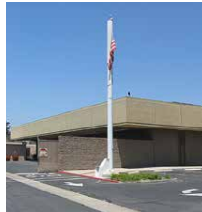
Copyright © 1997-2016 CellTowerPhotos.com. Used with permission.
