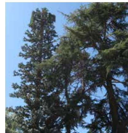
The above two faux trees above have needle coverings and natural-looking shape and dense foliage that blends with landscape context.
