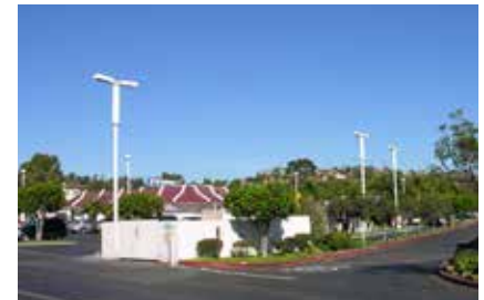
Copyright © 1997-2016 CellTowerPhotos.com. Used with permission.
