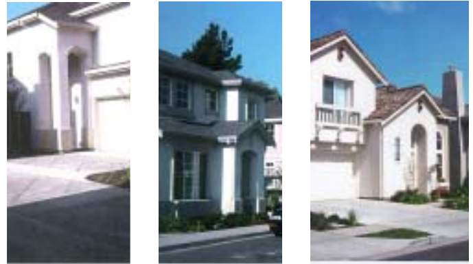
Undesirable Entries: Entries are frequently minimal and the homes lack the transition space between the street and living spaces as well as the architectural detail which porches can provide.
