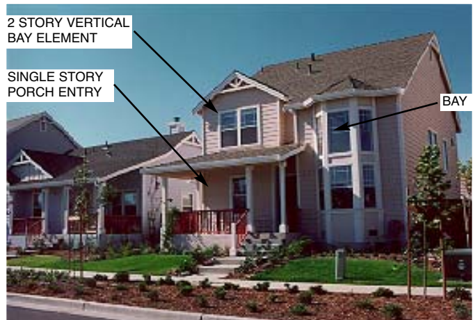
DGL 3.1.3: Each two story home shall have a vertical element to its massing, such as a two story entry feature, bay, corner turret or dormer, etc.
