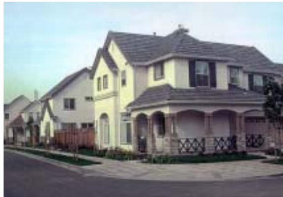
Desirable Corner Entry porch and Facade Design
