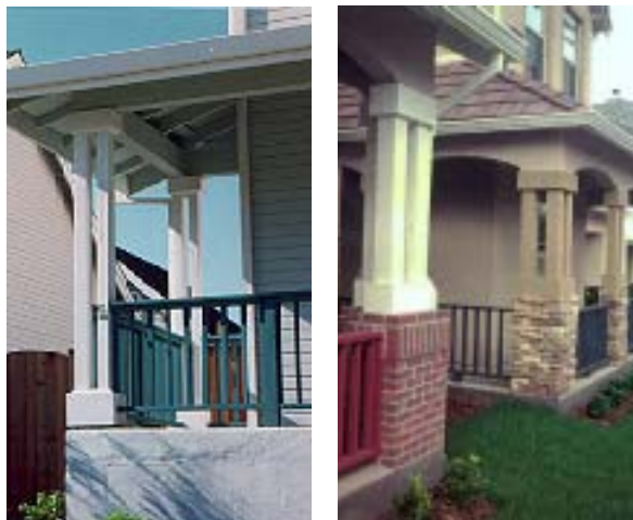
Desirable: Porches provide added architectural character, provide transitions and buffers between the street, living spaces and activity areas.
