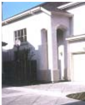
POORLY PROPORTIONED ENTRY COLUMN
