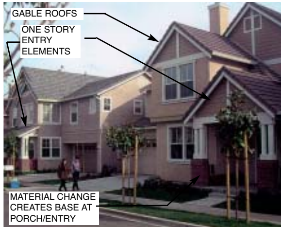
Desirable: High pitched gable roofs add vertical proportions and articulation to home facades.
