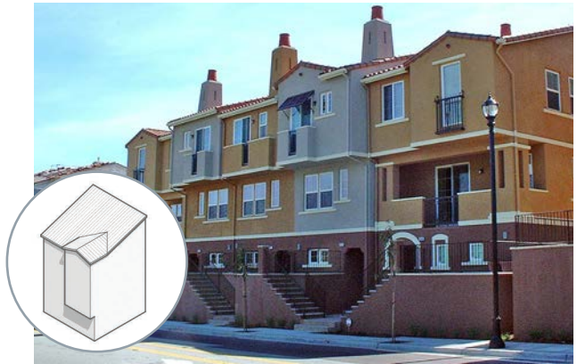
NOT RECOMMENDED - Bays should be distinct or set within main facade, not flush with side facades.
