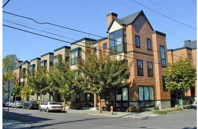
RECOMMENDED - Taller massing defines building features such as corners that create building articulation to reduce monotony.
