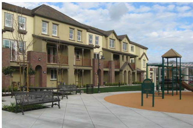
The key issues for these guidelines revolve around creating infill development that must consider both existing and planned interests when creating new development.
