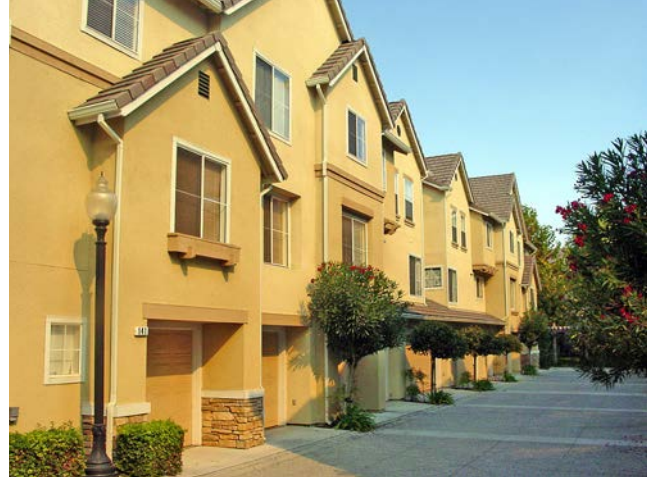
RECOMMENDED - Garage doors should be of a high quality and recessed. Material, pattern and color should be consistent with overall style of the building.
