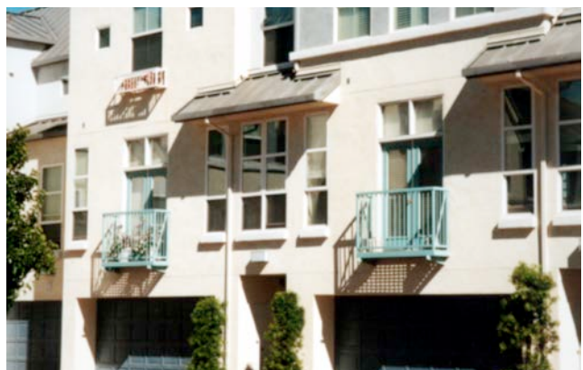
NOT RECOMMENDED - Balconies that are unusable because of their insufficient size.
