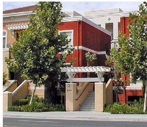
RECOMMENDED - Accents such as trellises, gates or arbors can be used to provide visual interest and demarcation to entrances.
