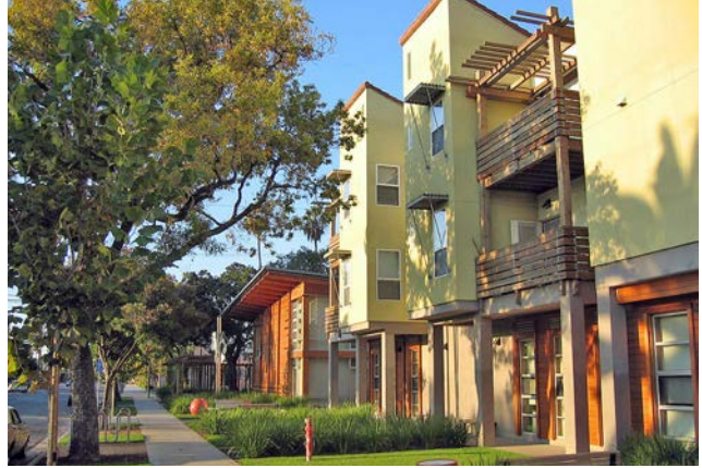
RECOMMENDED - Trellis and column material and proportions should be designed compatibly with project architecture so as to not appear applied to the building facade.
