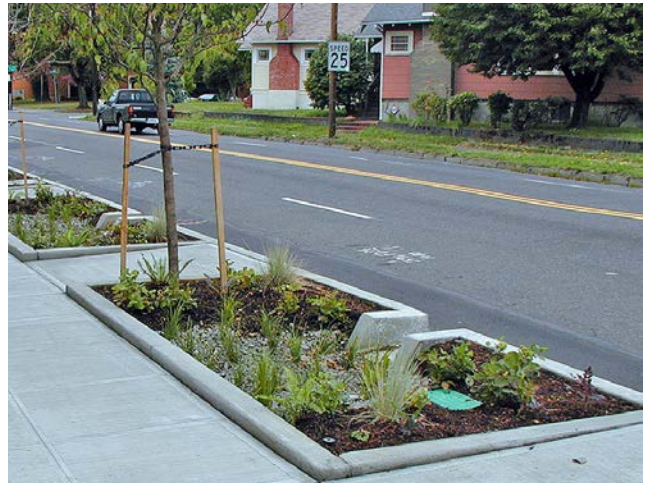
RECOMMENDED - BMP stormwater treatment facilities should be used to treat stormwater runoff.
