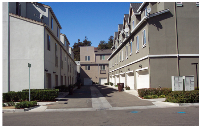
NOT RECOMMENDED - Building massing which dominates an auto court or private street without landscape relief creates "canyon effects."
