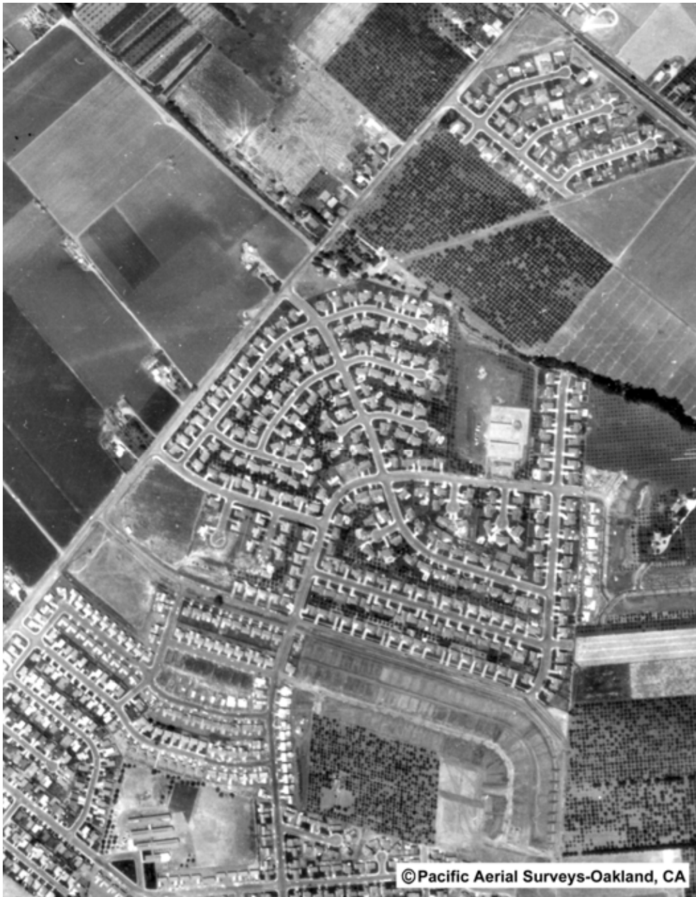
FIGURE 25. Mission Ranch, July 7, 1960. No more than a dozen of the 282 lots in the first five tracts are still vacant. Beyond Covington Drive, work is underway on the 36 houses of the final unit, Tract 2030 (right), where construction started two month before. Adjoined by Mission Ranch houses, Chadbourne Elementary School (right center) is ready to open. Mission Valley has made contact with Mission Ranch, and the first-ever segment of Paseo Padre Parkway is being laid out between the two subdivisions. (Courtesy of Pacific Aerial Surveys.)
