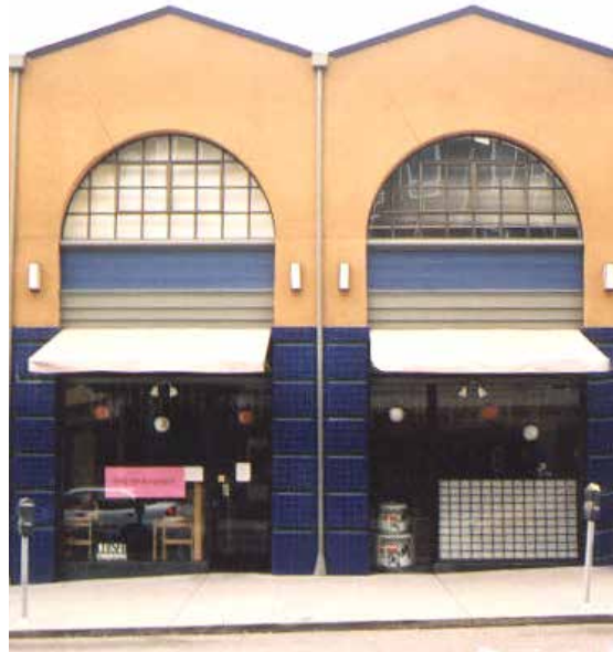
Example of awnings within structural bays.
