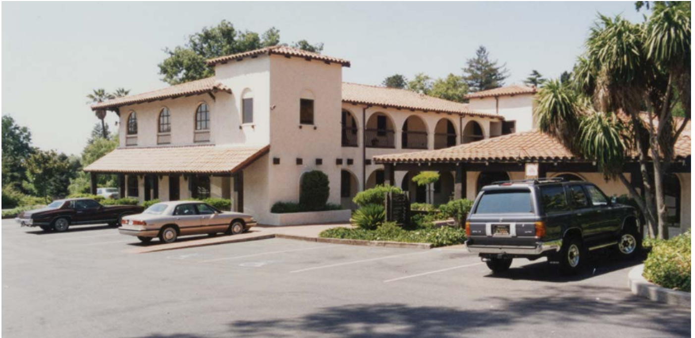
Figure 25. A stair tower provides visible access to office space on both the first and second floors of this Mission Revival style building.
