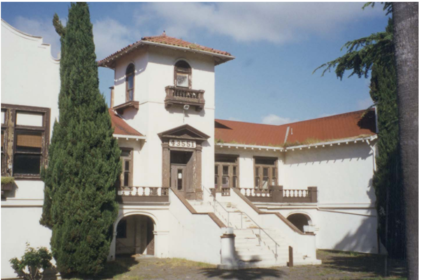
Figure 23. 43551 Mission Boulevard. The Old School building is a good example of the Mission Revival style.
