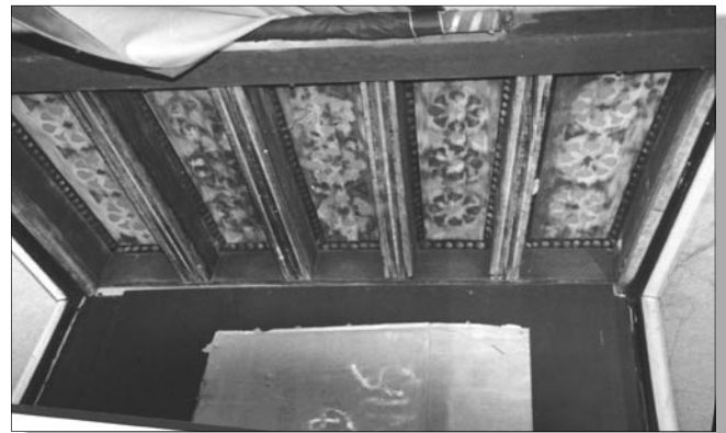
Figure 29 Decorative brick, tile, and painted coffer ceilings on commercial buildings in Niles
