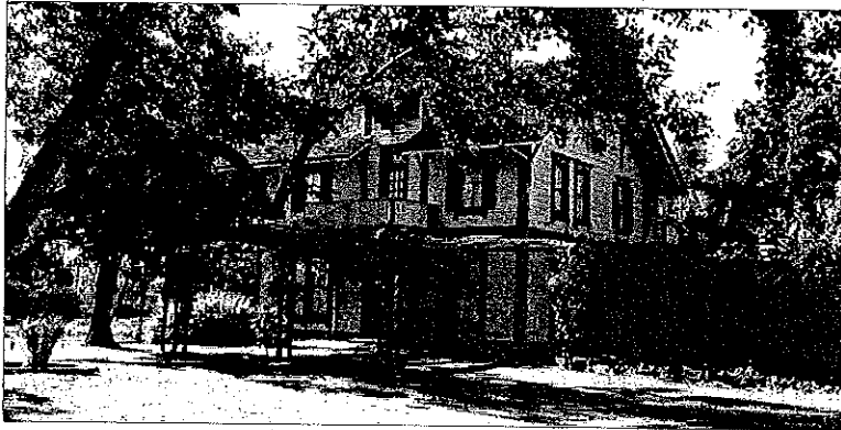
Fremont's historic resources offer unique opportunities to highlight the City's cultural heritage.
